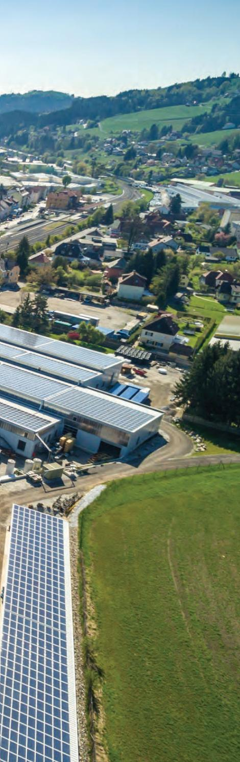
an area of 28,000 m<sup>2</sup> on the plant grounds. In addition, Bauer completely renovated the roof structures of the production halls and outfitted them with a photovoltaic system with a capacity of 2.3 megawatts. The system has been in full operation since December. This allows Bauer to produce 100 percent of the electricity annually at the Voitsberg site, making it independent in terms of its electricity supply.
