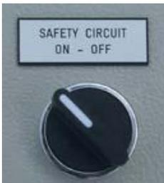
7. Turn the "SAFETY CIRCUIT" switch to "ON".
