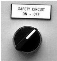
1. Turn the "SAFETY CIRCUIT" switch to "OFF".
