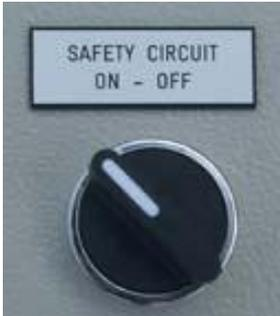
6. Turn the "SAFETY CIRCUIT" switch to "ON".
