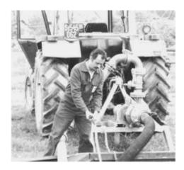
Engage the PTO, run up at low engine speed, and open the foot valve of the suction line.
