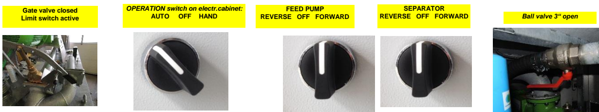
Figure 20 lever and switch position in Automatic operation with clear effluent pump
