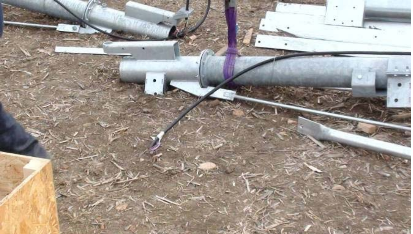
Installation of the bracket and clamp for fastening the drive tower legs to the main pipe
