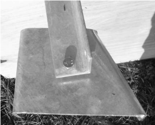
Installation of the brackets L and R on the overhang struts.
