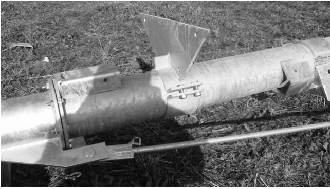
Overhang clamp installed
