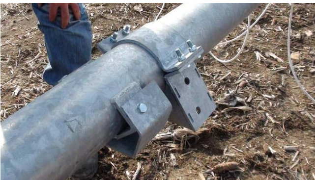
Installation of the bracket and clamp for fastening the drive tower legs to the main pipe
