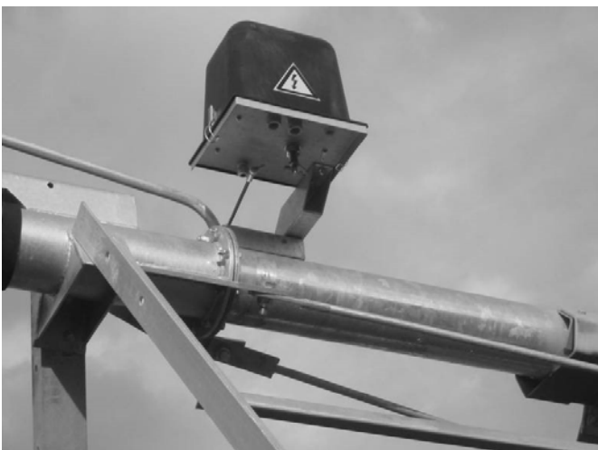
Alignment box installed.
